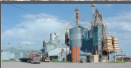
Commercial Grain/Livestock Feed Facility
